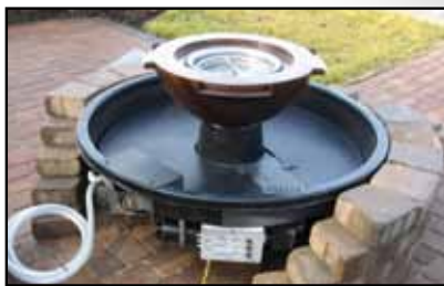
360 Feature being finished with paver stone
